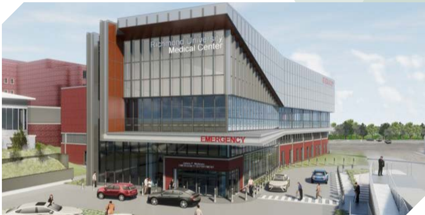
RUMC's new Emergency Department, scheduled for completion next year, was one of many capital improvement projects highlighted during this year's gala.
