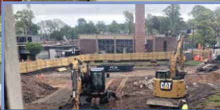
NEW EMERGENCY DEPARTMENT UNDER CONSTRUCTION
